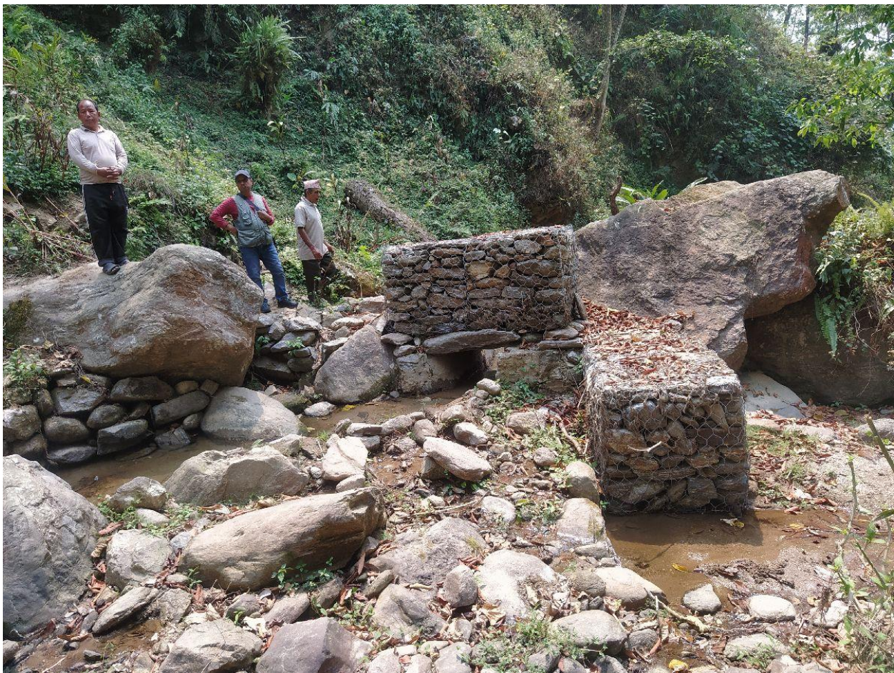
Annex Photo 15: Intake of Khung Khola Titriya Sejepa Phewadin IS in Panchthar.
