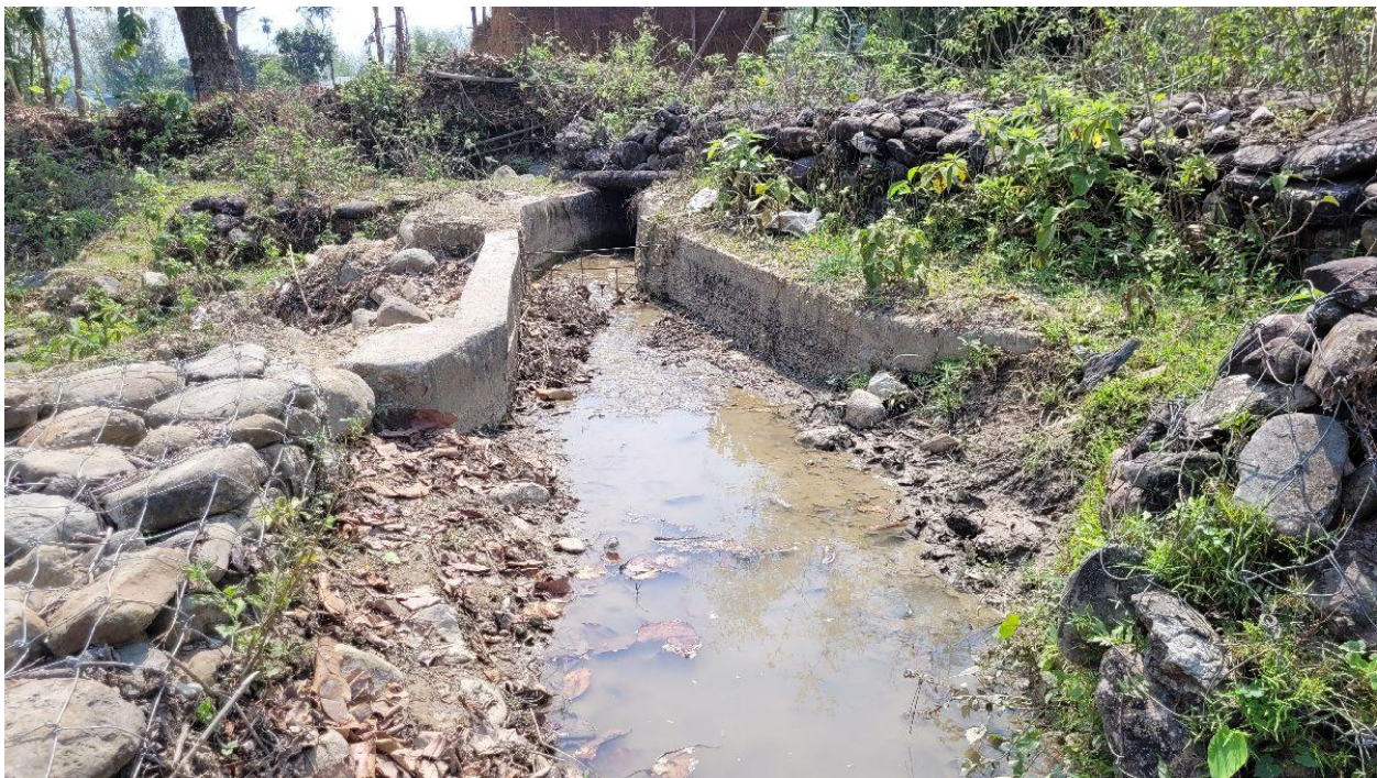
Annex Photo 3: Intake of Katari Sinchai Yojana IS.
