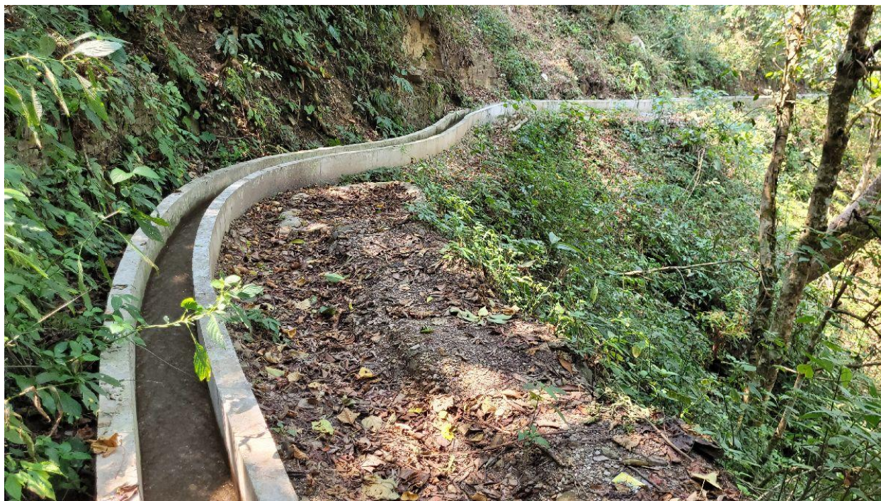
Annex Photo 4: Canal RCC lining in Pakhale Khola Dhonde IS.
