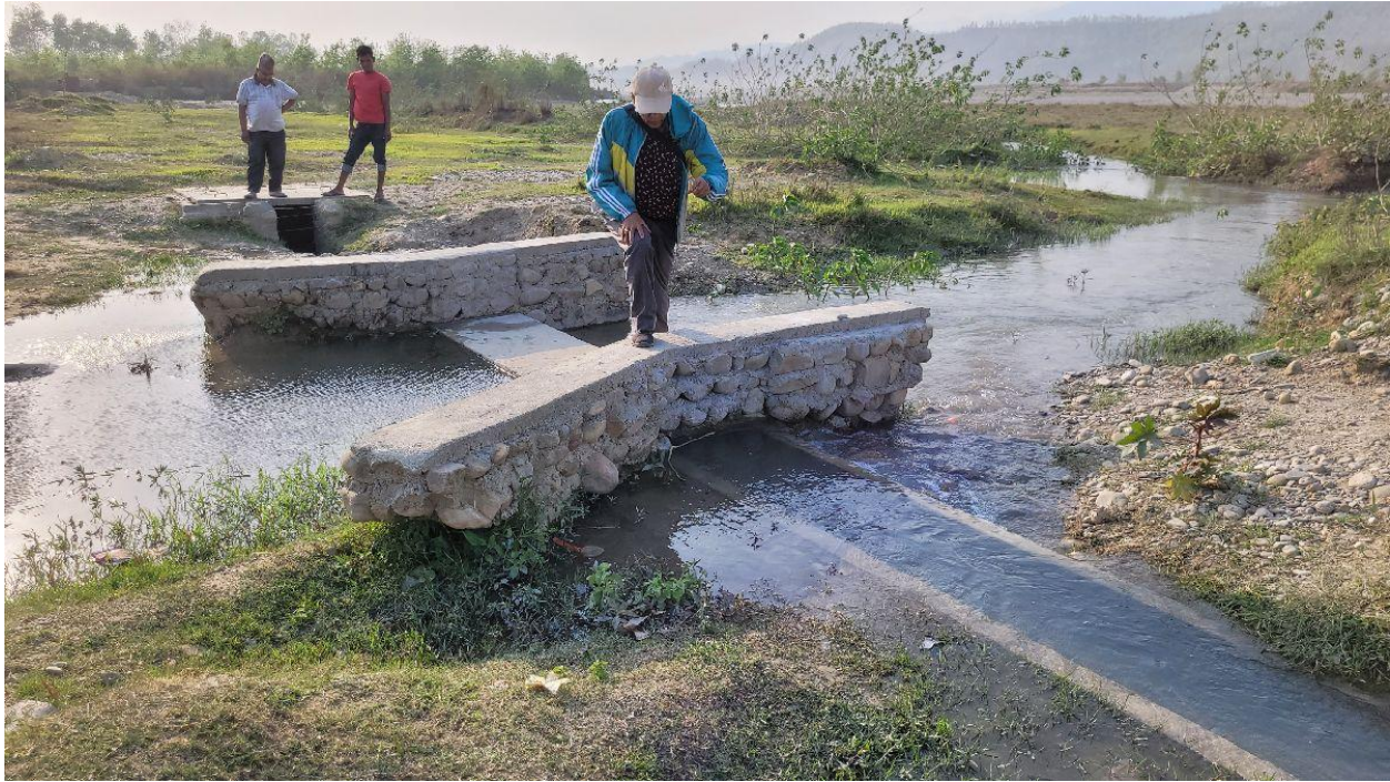
Annex Photo 1: River crossing structure in Hadaiya Sana Sinchai Aayojana IS.
