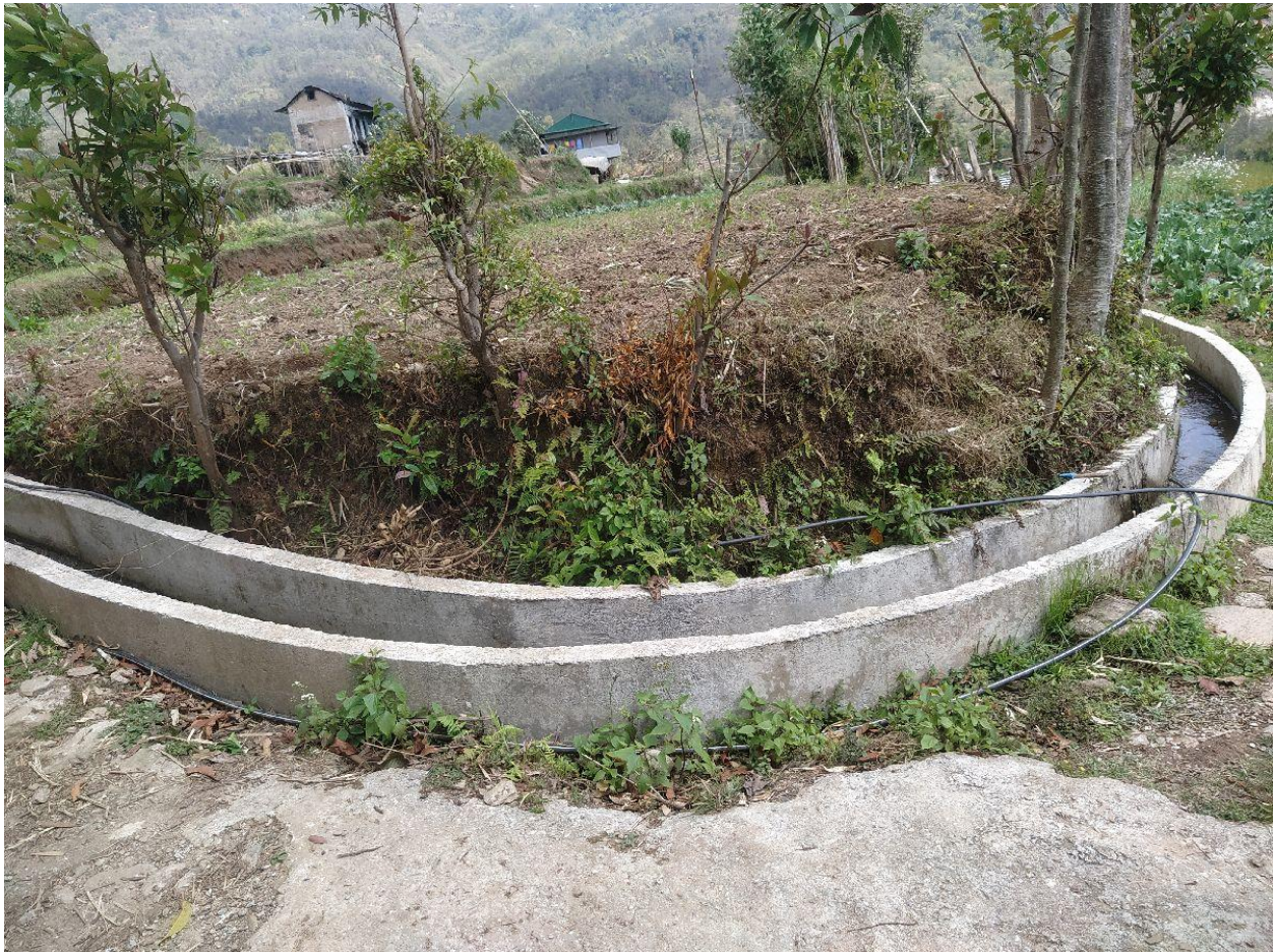
Annex Photo 10: Canal lining in Argeli Taksar IS in Okhaldhunga.
