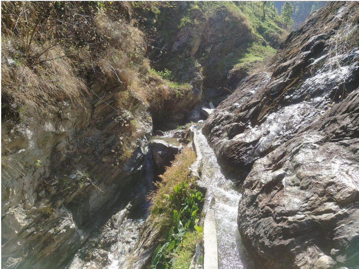
Annex Photo 11: Main canal in Andheri Rupse IS in Okhaldhunga.
