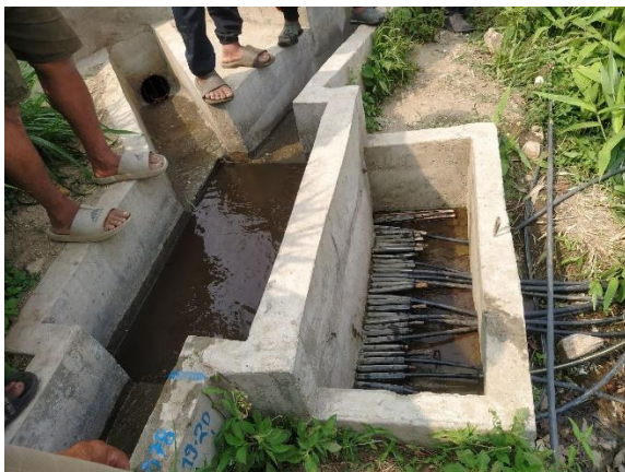
Photo 3-4: Individual farmers using small pipes for sprinkler irrigation, needs appropriate design for distribution pipes for sprinklers.
