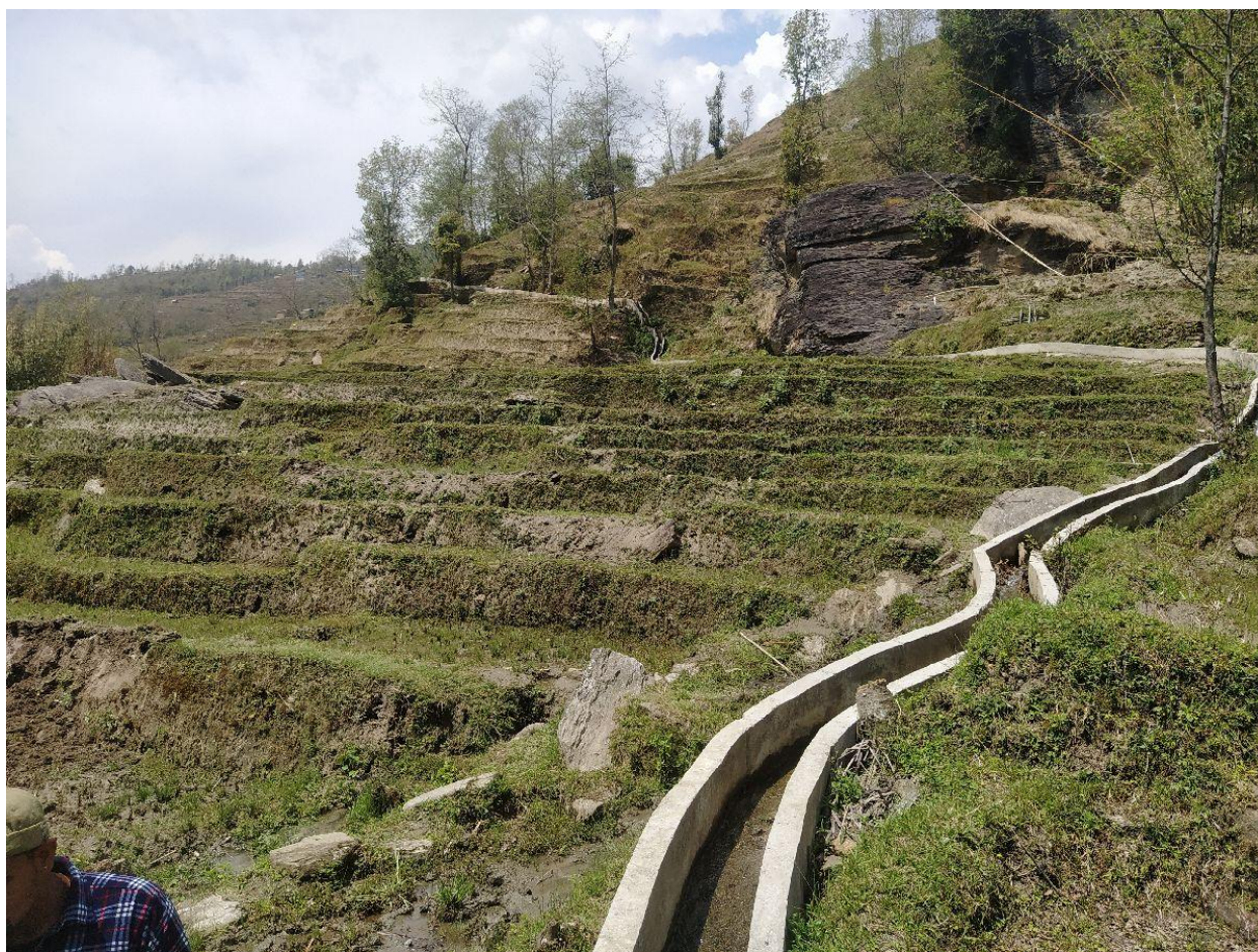
Annex Photo 7: Canal lining and command area of Jaljale Chuchhe Dhuna Dobela IS in Khotang District.
