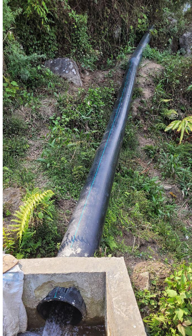
Annex Photo 6: Pipe conveyance in Taname IS, Tehrathum.
