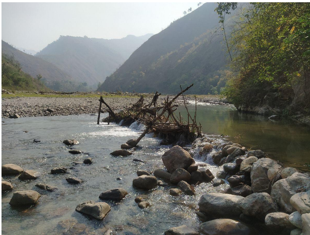
Annex Photo 12: Temporary diversion from the river to intake in Kabre Mahabir Sichai Yojana IS in Okhaldhunga.
